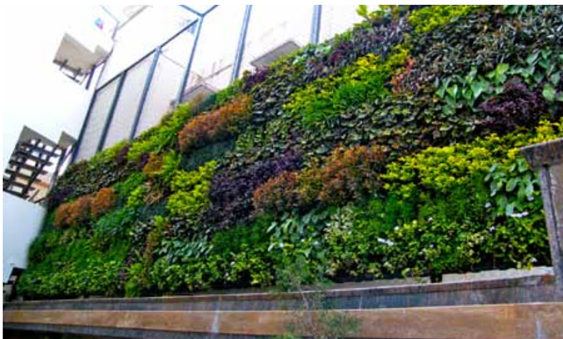
Compound Wall, Bengaluru. Photo: Courtesy of ELT India
